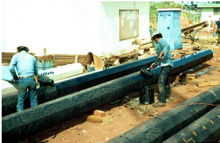
Fig. 7.45 View of applying a bitumen coat to a concrete pile
