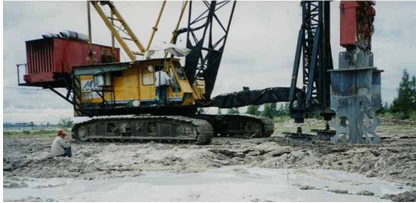
Fig. 10.16. Liquefaction of water-saturated sand during the initial phase of compaction. Note that water has collected on the ground surface. The original groundwater table was 4.5 m below the ground surface.
