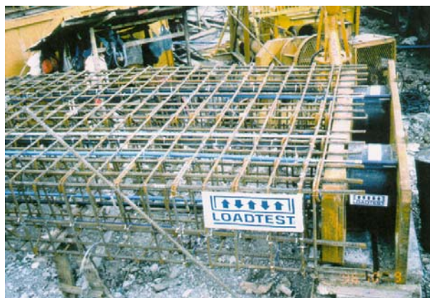
FIG. 2. O-Cell Assembly and Reinforcing Cage
