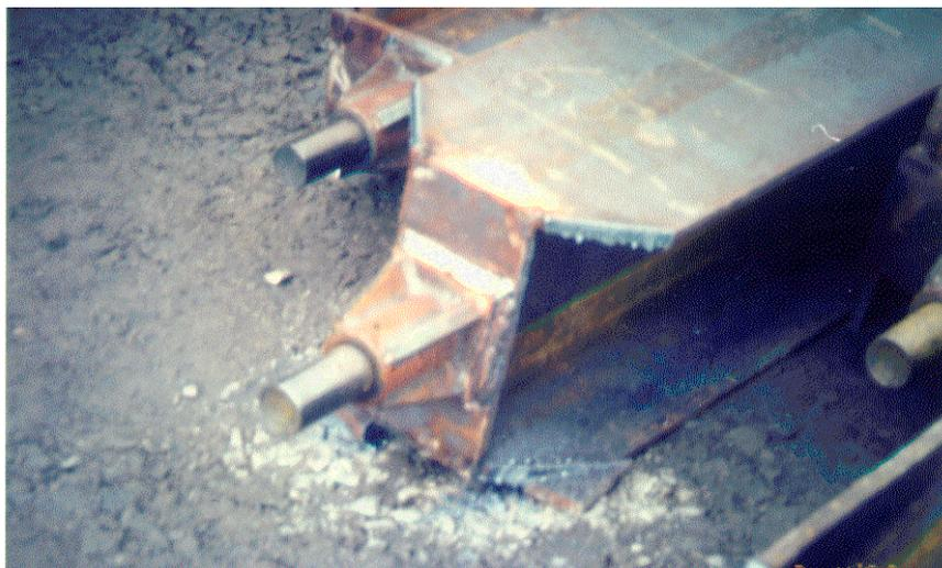
Fig. 6a H-pile with the Herkules rock shoe attached
