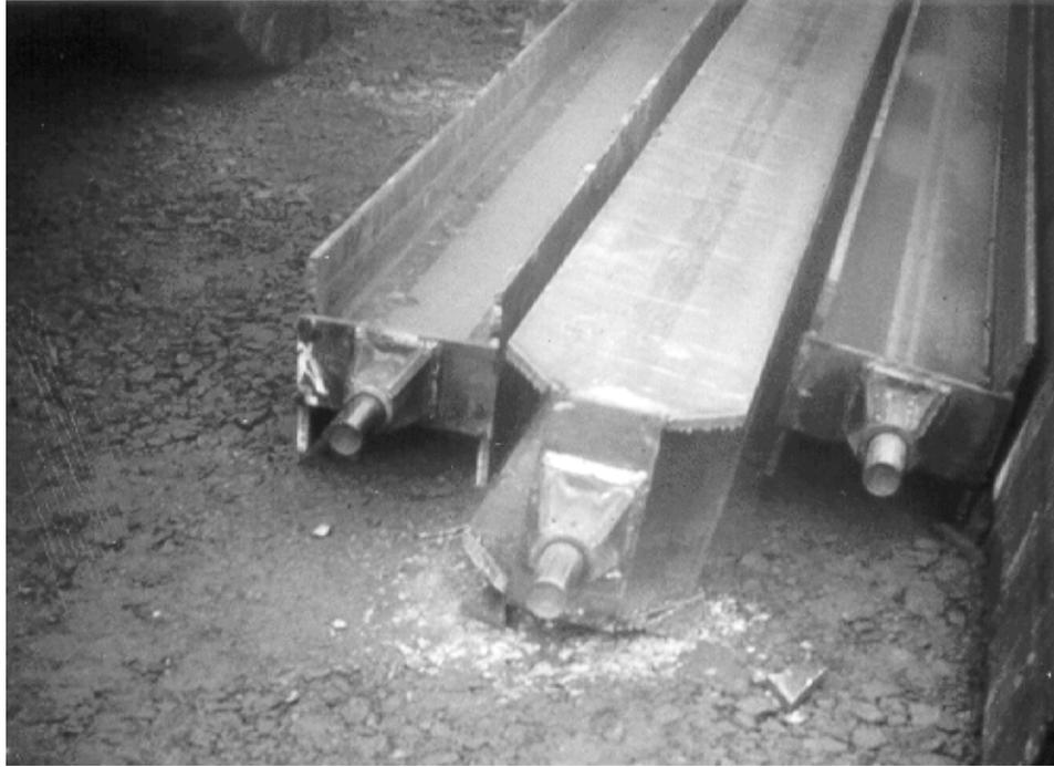
Fig. 6b H-piles with the Herkules rock shoe attached ready to be driven
