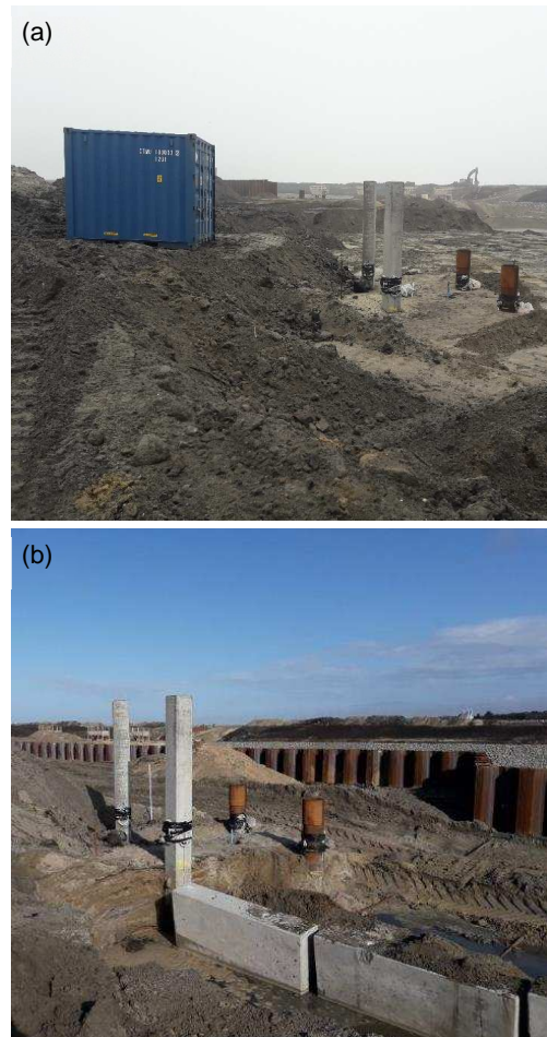
Figure 6. Test site at (a) Day 78 and (b) Day 126 (before placing the 3.0 m fill). The concrete slabs in (b) are anchor plates for the sheet pile wall seen in the background.
