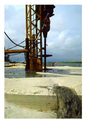
**Figure 4.** Water flow as evidence of liquefaction during compaction of the hydraulic fill inside the concrete caisson (source: Massarsch and Lindberg, 1984)
