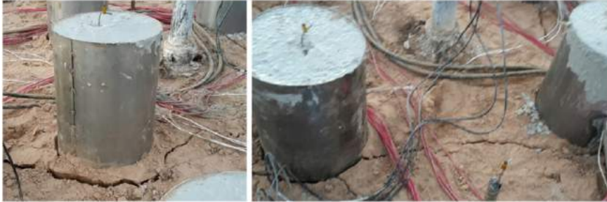
Figure 13. Photographs of cracks in ground surface at a corner pile and at two side piles.
