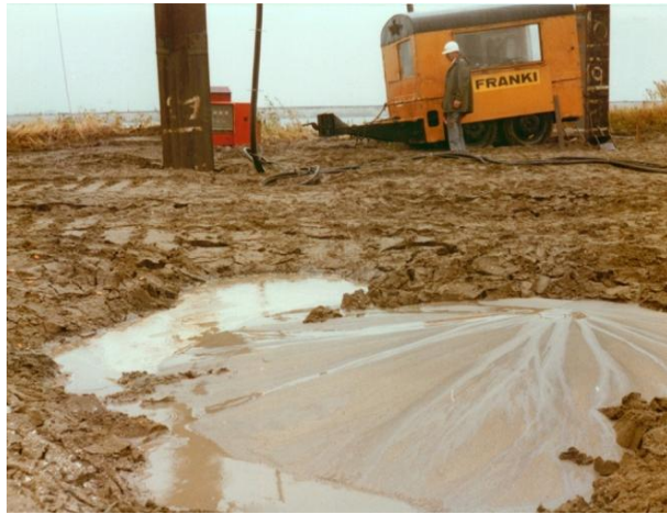
Figure 1. Liquefaction caused by TriStar soil compaction at Borechem (Wallays 1982).
