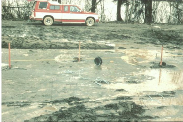
Figure 6. Settlement in the compacted zone, averaging 0.3 to 0.45 m. A zone of soil liquefaction is apparent in the right of the picture.
