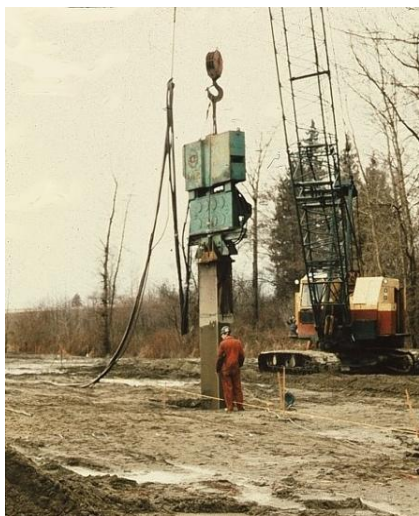
Figure 3. Resonance compaction at Annacis Channel, Vancouver by TriStar probe with variable frequency vibrator.
