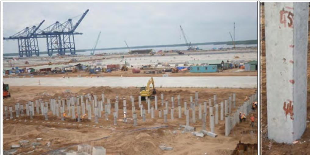
Fig. 10. View on Feb. 10, 2012, of the Maintenance Shop area with about half the piles lengthened (Authors' photo)
