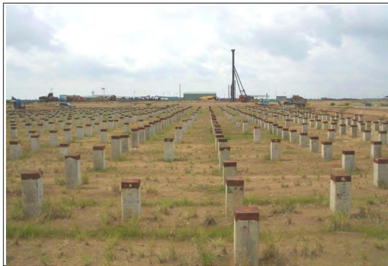
Fig. 15 View on October 4, 2011, from south end of CFS building showing some of the about 750 piles driven for the CFS building (Authors' photo)
