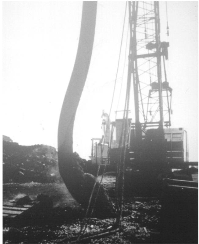
Fig. 4b Doglegged pile during extraction
